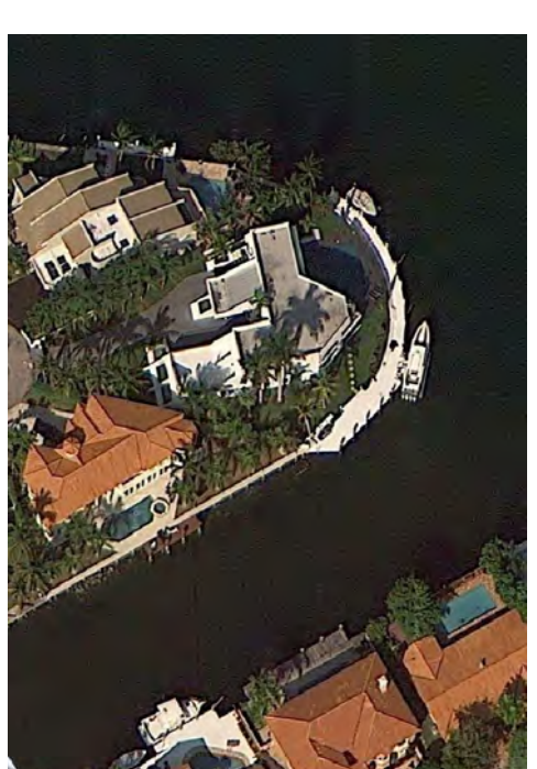
HOUSE 9 (Roof top terrace)
