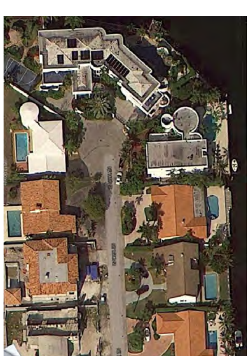
HOUSE 4 (Roof top Terrace)
