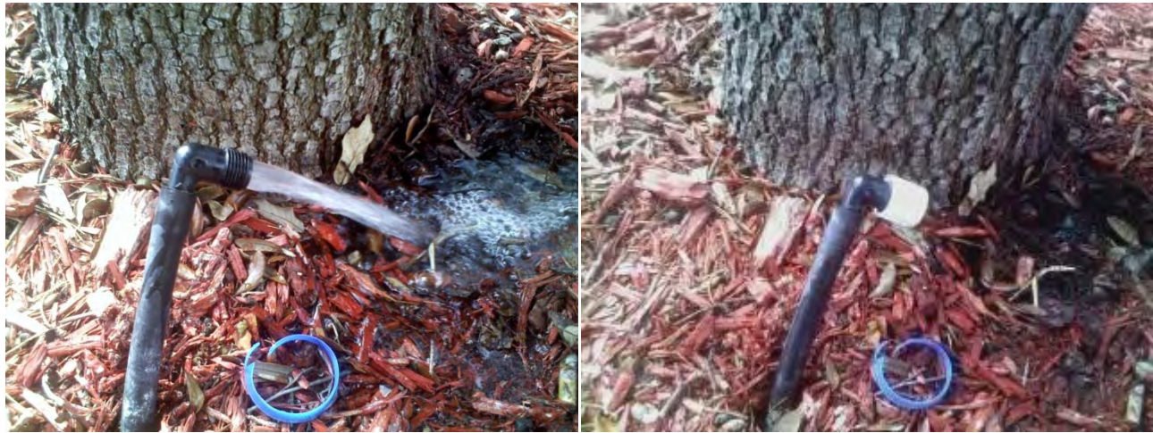
Repaired six irrigation systems; 120 heads installed; laid 308 linear feet of pipe
