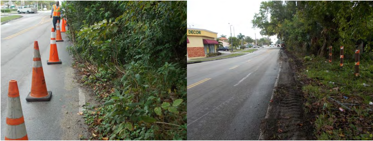
Improved roadway clearance at West Dixie Hwy. 172 nd Street
