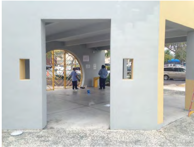
Performed five major paint requests
